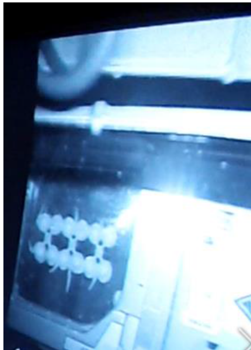
Fig. 1. Image from the internal cameras in the EMCS, drawn from the live video screen in the control room. The loose water cable is visible in the top left corner
